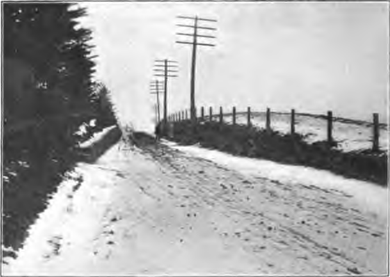
New Brunswick and Bound Brook road, Middlesex Co. Landing Hill, during improvement.
